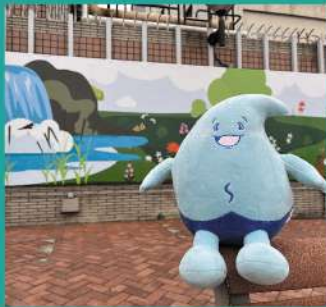
Sheung Wan Salt Water Pumping Station
