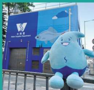
Tong Shui Road Fresh Water Pumping Station
